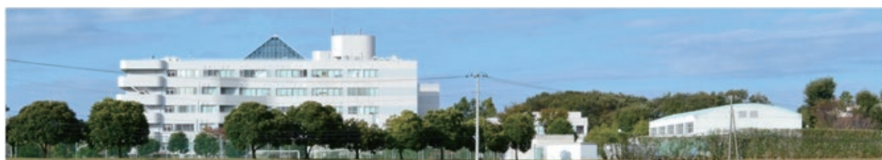
天久保キャンパス校舎棟 School buildings in Amakubo Campus
